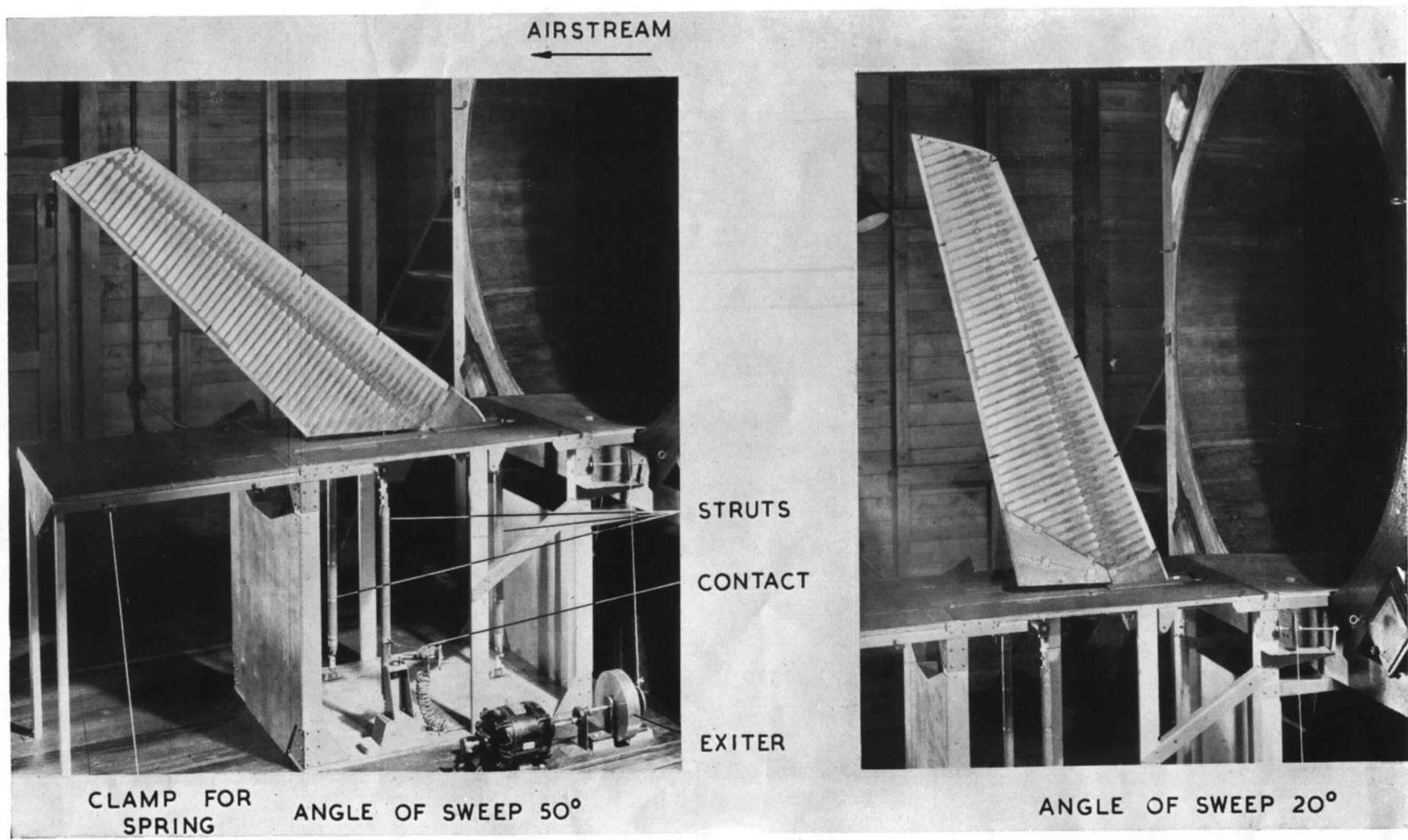
FIG. 1. Flutter Rig in Wind Tunnel.
